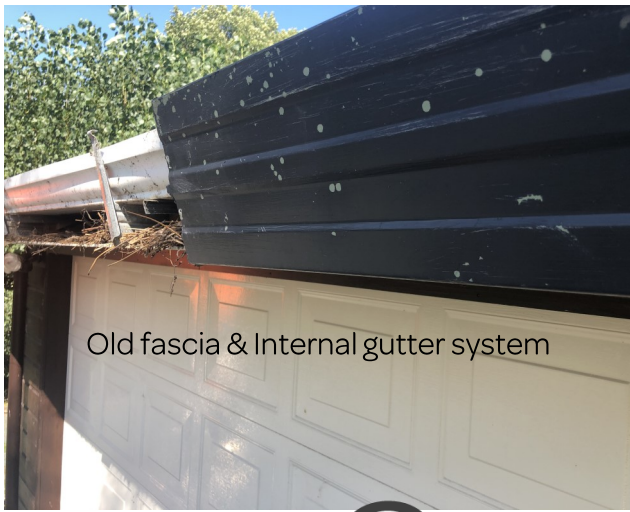
New Conform fascia ready for external gutter
